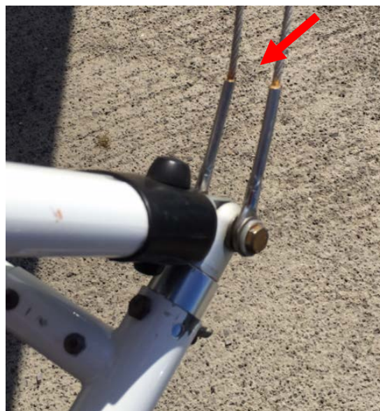
Fig 2. Overall general arrangement of the GT450 lower side rigging cables with roll-swaged terminal ends. The arrow shows the point of partial failure. The attachment bolt at the control frame knuckle should be just loose enough to allow each cable to align with the load. Note the plating on the bolt head is shiny in this example.
